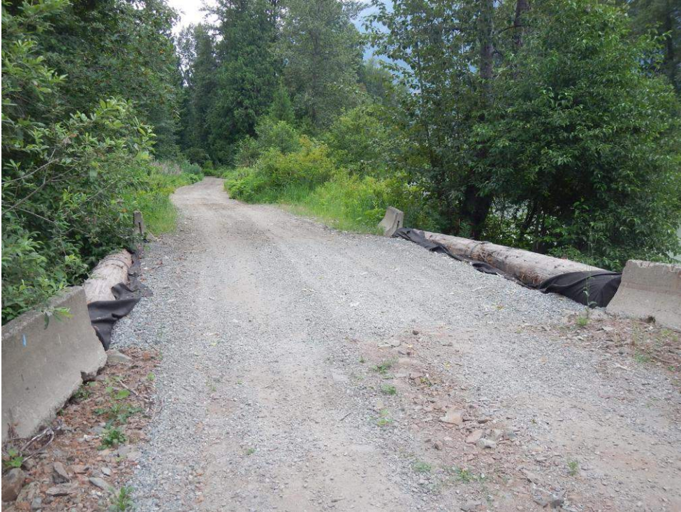
2.6 km recently replaced 6 metre long bridge
