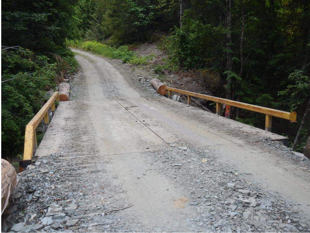
3.6 km a major 9 metre bridge recently replaced
