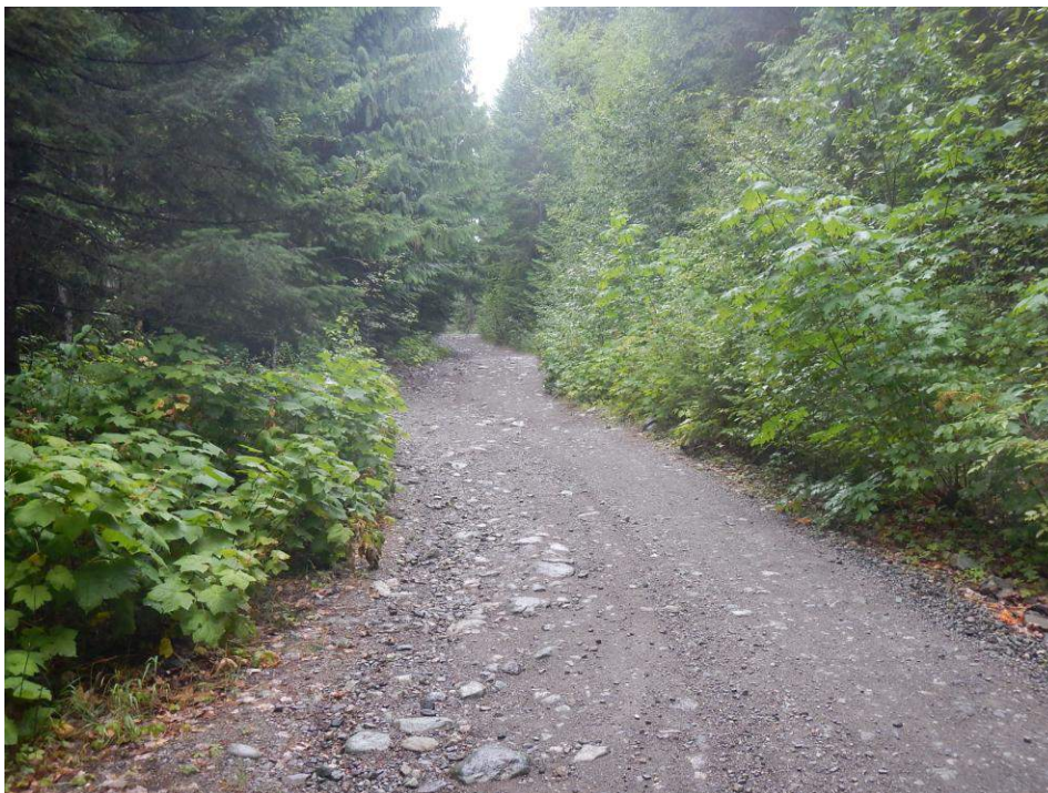
3.8 km steadily climbing road. Could use more and better water bars
