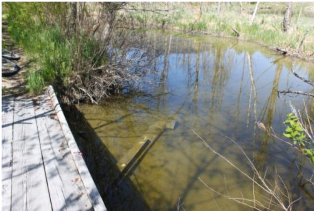
Figure 3. Pipes installed through beaver dams at the inlet to the lake.
