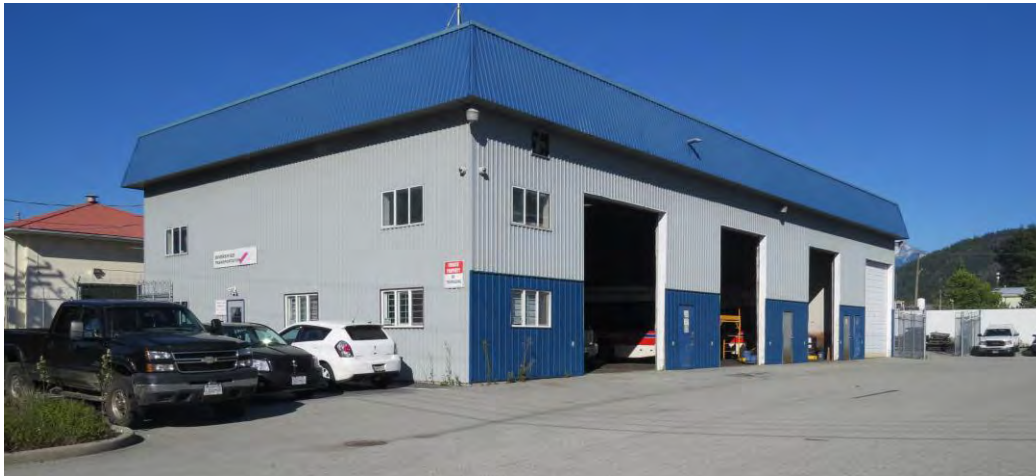
Figure 32: Squamish Transit Garage.
