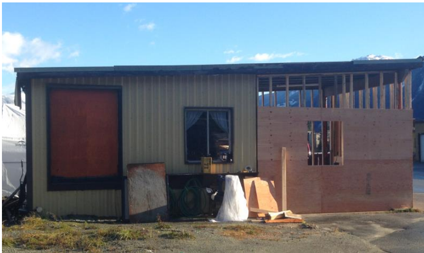
Tool Shed Addition, October 2015
