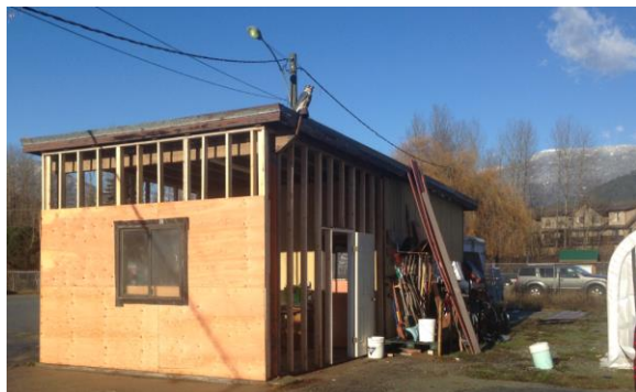
Tool Shed Addition, October 2015
