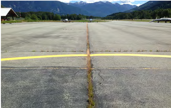
Large traverse cracks on apron
