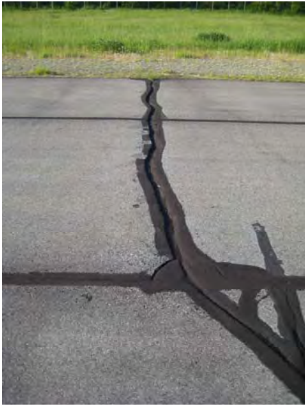
Large traverse cracks on apron
