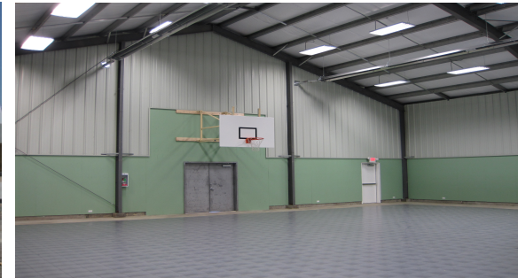
A pre-engineered metal building with sport flooring and plywood panels to protect metal walls
